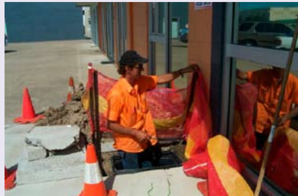
Installation of Dark Fibre
